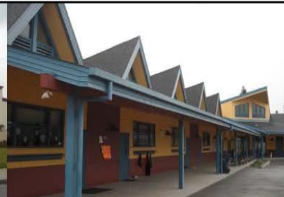
2004 Booksin Elementary Classroom Building
