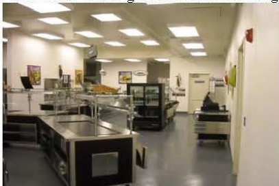
2009 Leland High School Kitchen Renovation
